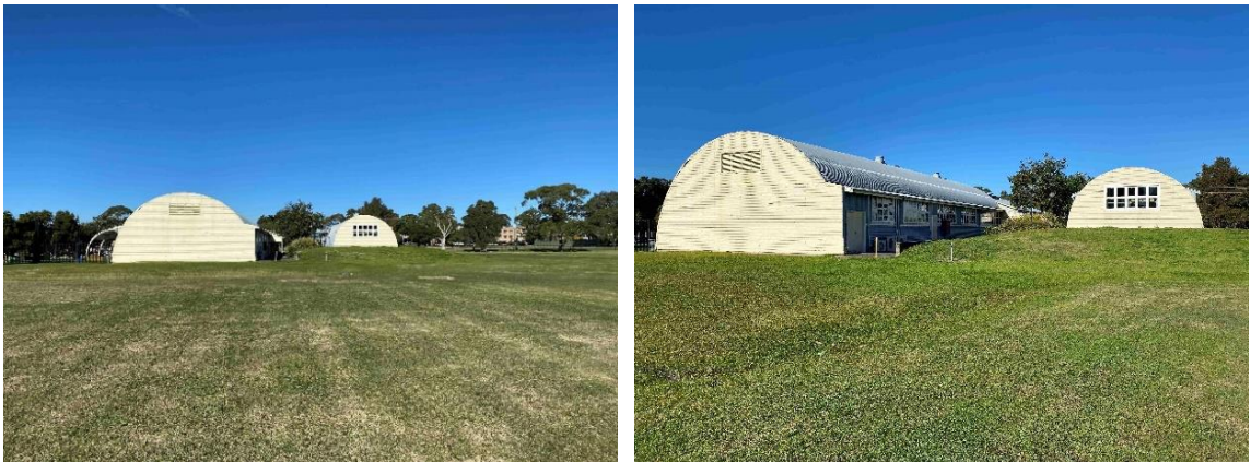
Buildings 201 and 204 viewed from the North
