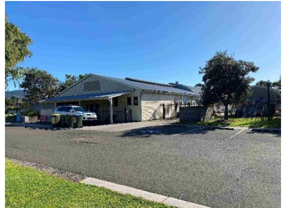
Building 201 viewed from the South East
