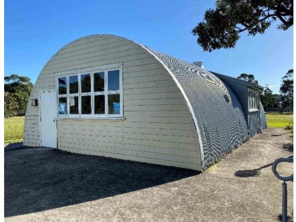
Southern facade of Building 204
