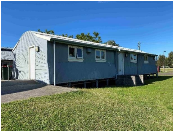
North and West facade of Building 210
