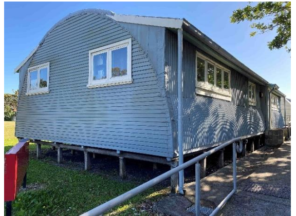
South facade of Building 210
