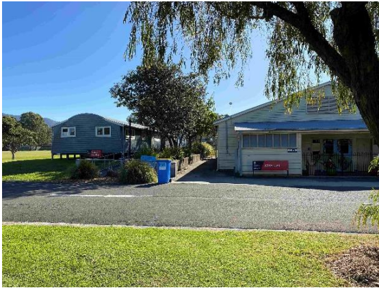
Buildings 210 and 201 viewed from the South
