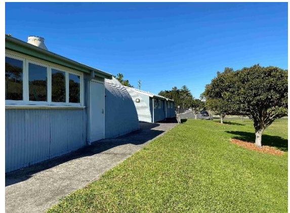
Buildings 204 and 210 viewed from the North
