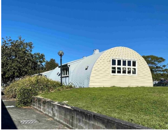
North and East facade of Building 204
