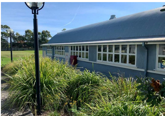
Western face of Building 201
