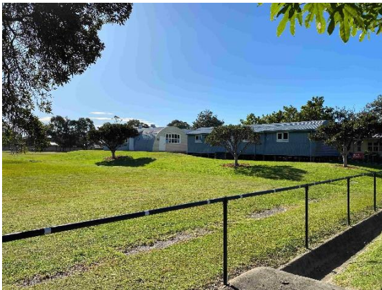
Buildings 204 and 210 viewed from the South West
